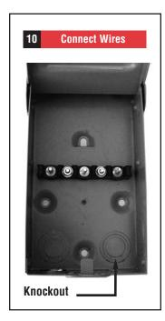
10. Remove the knock out in the lower right corner of the external connection box. From the rear of the connection box, feed wires & 4 pin plug into box. Slip the lock nut over wires and plug and tighten securely onto conduit coupling. Connect the black, red, and white wires to separate threaded lugs and tighten securely. Screw the green ground wire securely to the bottom of the box. NOTE: THE 4-PIN PLUG WILL not be connected to any mating plug or other wires.
